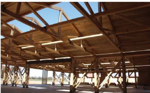
A view from inside the hangar
